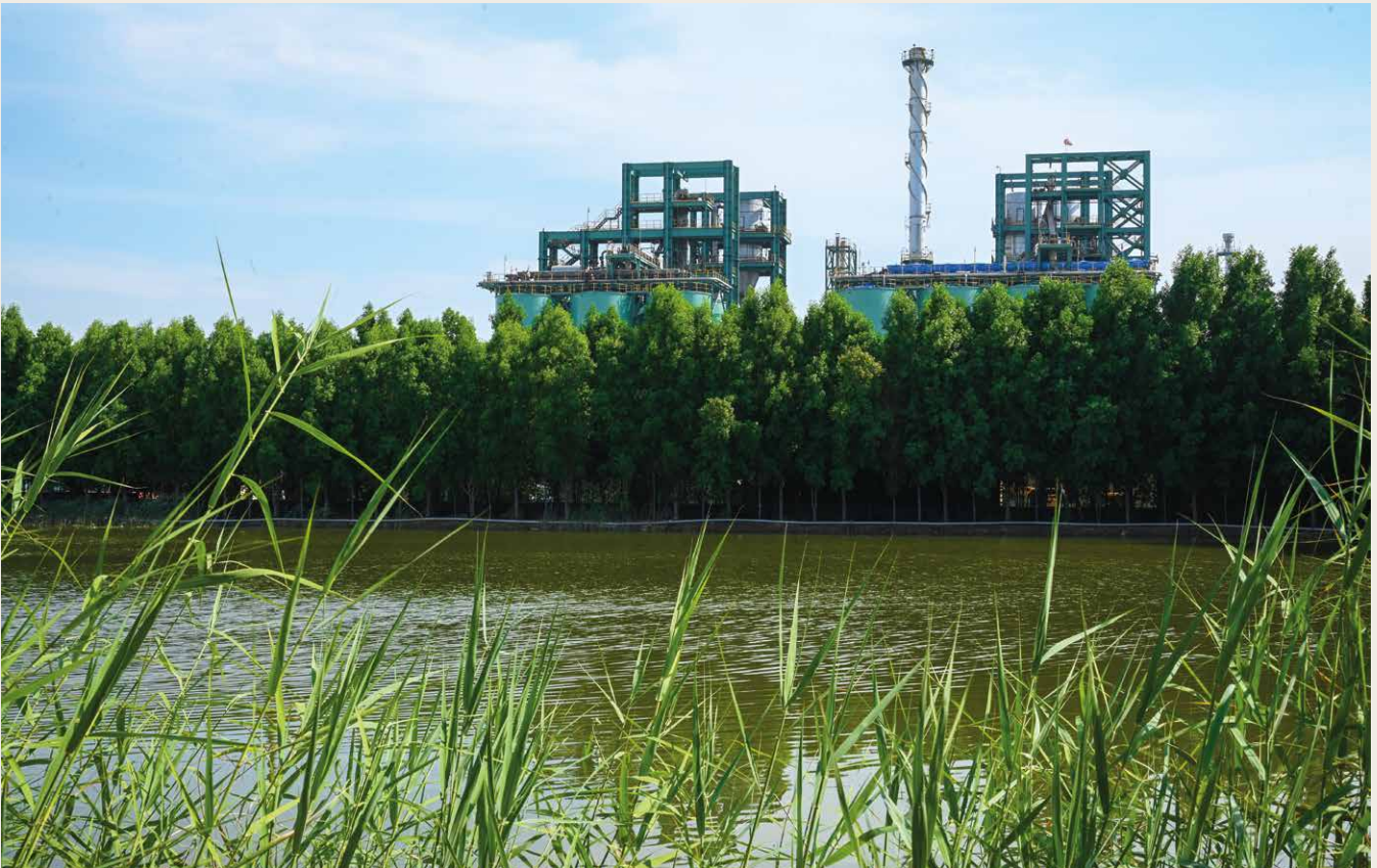
Rainwater Harvesting Pond
