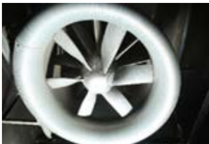
Air Handling Unit-Centrifugal blower replaced with energy efficient axial flow fan.
