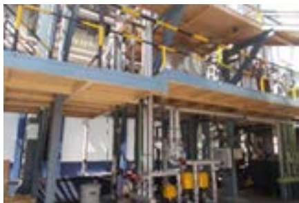
Installed new set up for deaerators at Chopanki site to use HI curing line dome flash steam.
