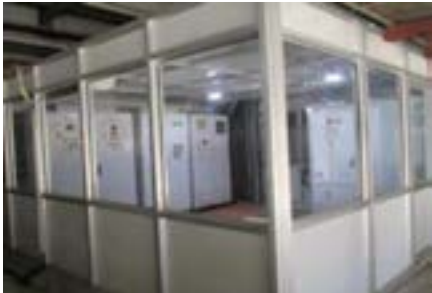
Installed live VFO panels in the utility section to replace Star-Delta starters, using PIO controllers for motor RPM control.
